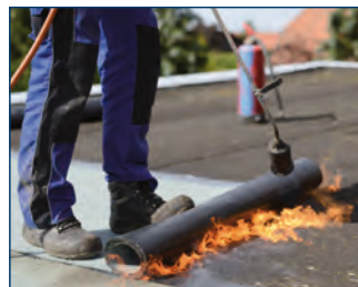
Bitumen carrier for roofing membrane
